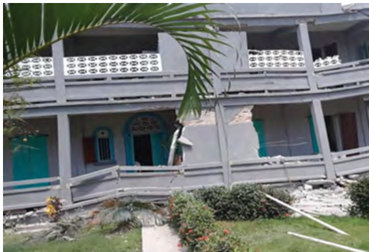
After the passage of the earthquake, the first floor spread out and flattened, giving way to the two floors. – Photo: Rosette Lafortune, M.I.C.
