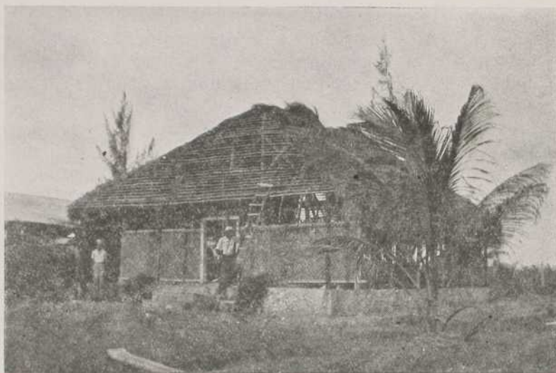
THE SCHOOL UNDER CONSTRUCTION AT CHARITY, IF YOU PLEASE . THE ROOF IS MADE OF BAMBOO STALKS AND STUBBLE. THE OUTER WALL IS OF BAMBOO TWIGS INTERTWINED.
