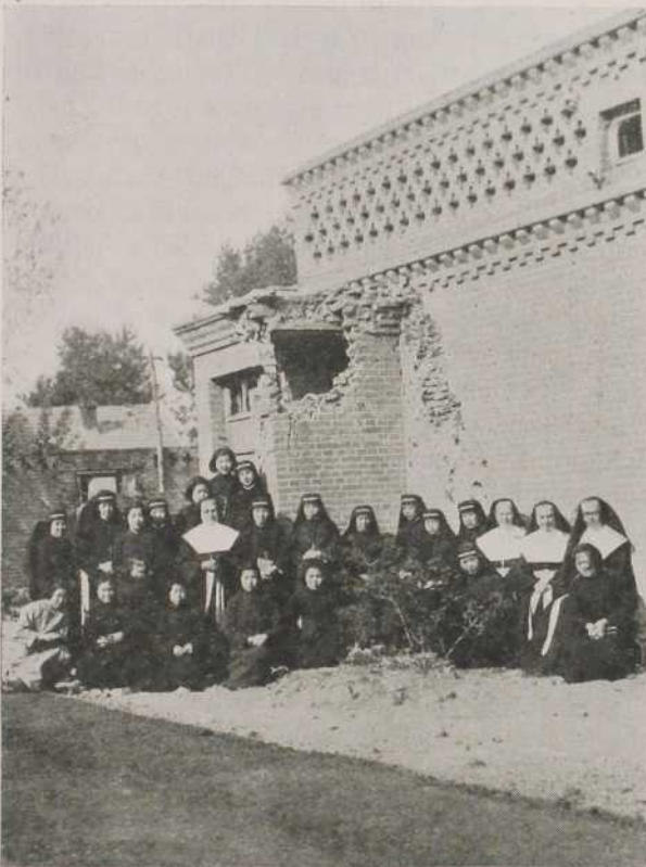
DAMAGES CAUSED BY A BULLET ON THE WESTERN SIDE OF THE FORMER APOSTOLIC SCHOOL OF SZEPINGKAI
