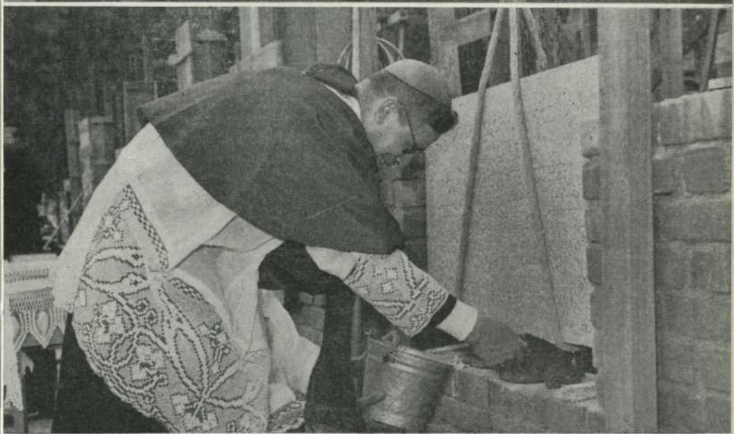
Above: Reverend Father Orlando, pastor of St. Teresa's parish, places the copper casket inside the stone.
