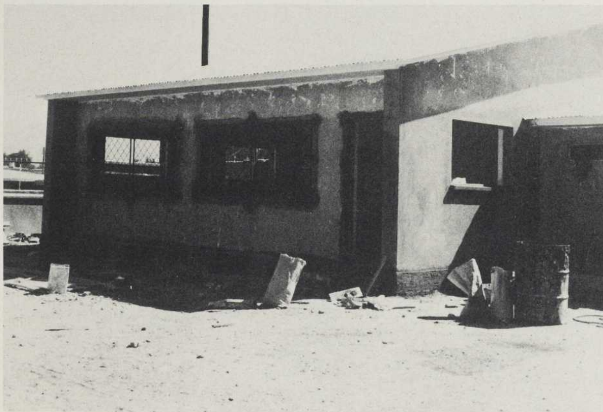
Construction of a workshop for the girls of Escuela Inmaculada Concepcion .
