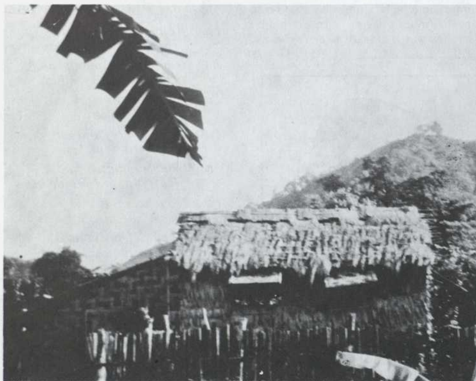
The fence which seems to isolate the Sisters is in reality an open door of welcome.
