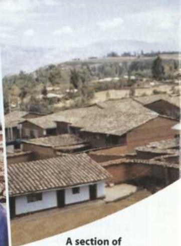
A section of Cajabamba village
